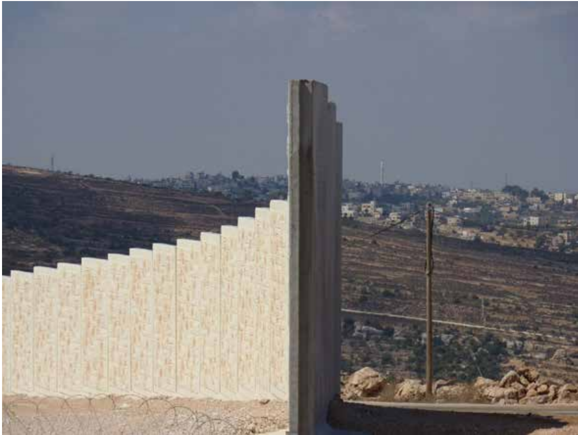
Figure 4. The Separation Barrier around al-Walaja under construction in 2010. This section separates al-Walaja from the Har Gilo settlement and Jerusalem beyond. The Palestinian side has been left in raw concrete. The Israeli side has been clad with a sandstone façade to minimise the visual disruption of the vistas of the expropriated lands of al-Walaja which have been designated as the Emek Refaim Park (Baillie 2013). © Baillie 2010.
